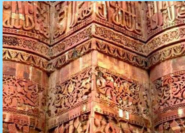
External Stucco work
