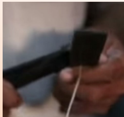
Pulling into wire
