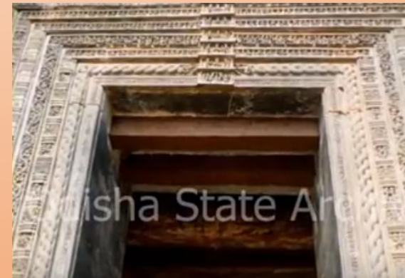
Beams in the door-way
