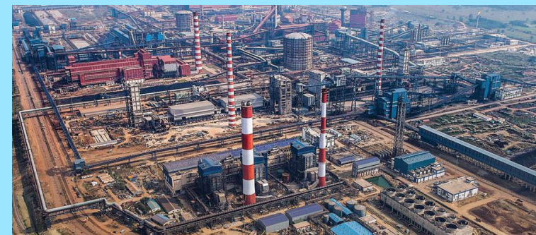
Tata Steel Plant, Jamshedpur
